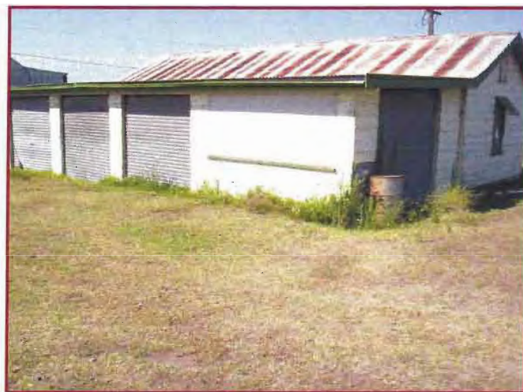
Photo 18 – Former dairy shed, looking south-east.
