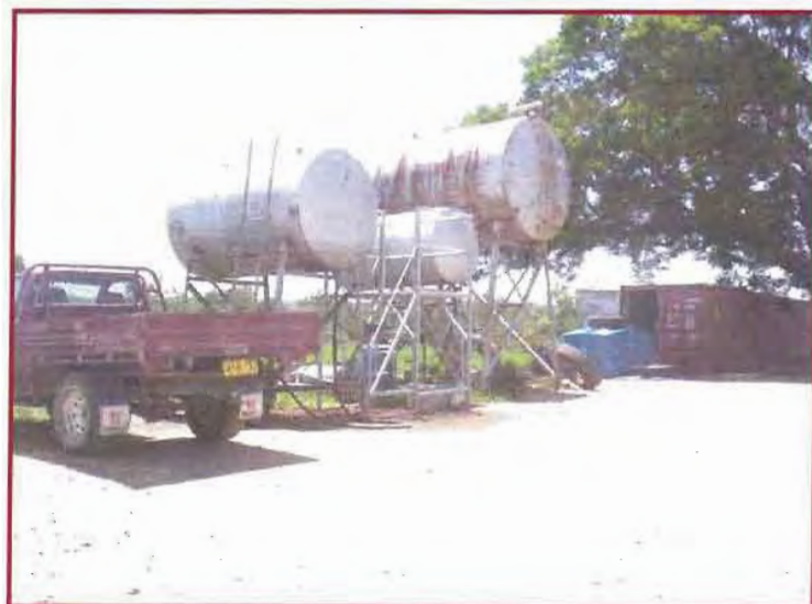
Photo 23 – Above ground fuel storage tanks located on the southern boundary of the site.
