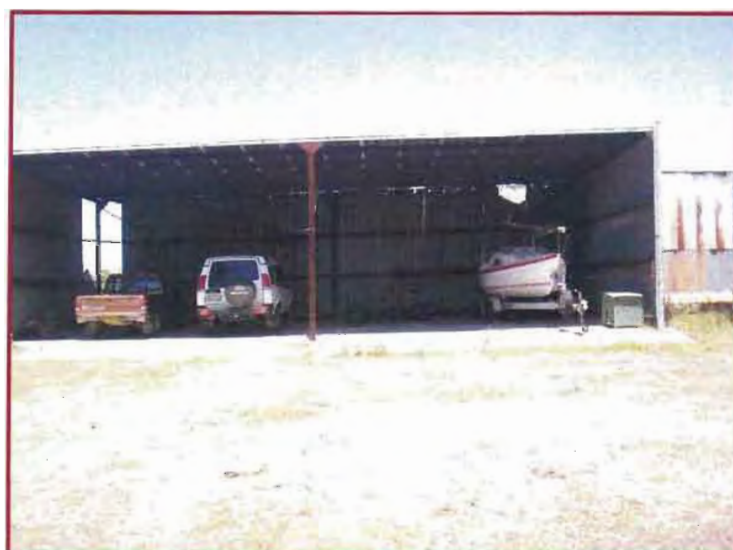
Photo 19 – vehicle storage shed, looking south.
